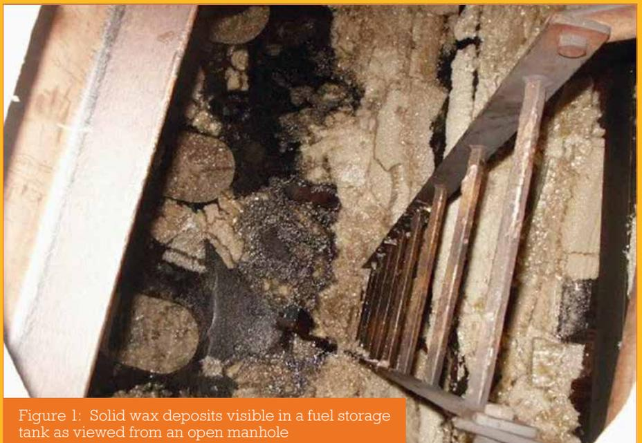
Figure 1: Solid wax deposits visible in a fuel storage tank as viewed from an open manhole
